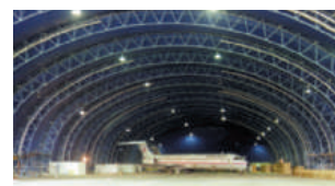
Airbus hangar, 1982 Germany — Précontraint® 1302 Resistance to traction after 22 years: Warp 97 % - Weft 84 %
