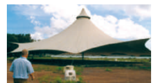
Exhibition marquee, 1982 Port Saint Louis — Précontraint® 1302 Resistance to traction after 18 years: Warp 86 % - Weft 76 %
